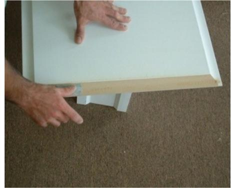
**Step 4** :: Tip- The MDF panels come unprimed, before installing panels on to the rails, prime edges first. For better results, you may want to prime and sand the edges twice. The face of the panel only requires one coat of primer.
